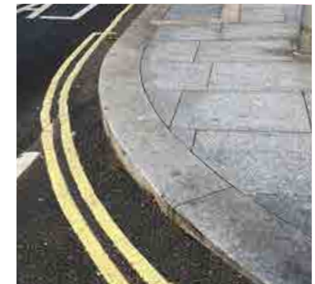
Granite kerbs will typically require less repair/replacement than concrete kerbs and will usually have a lower whole life carbon impact, when sourced sustainably
