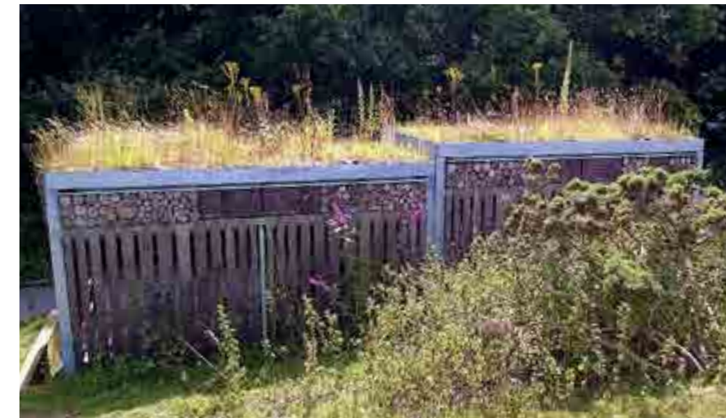
Purpose-built cycle shelter with green roof and timber cladding to blend into the surrounding landscape. Credit: Grass Roof Company
