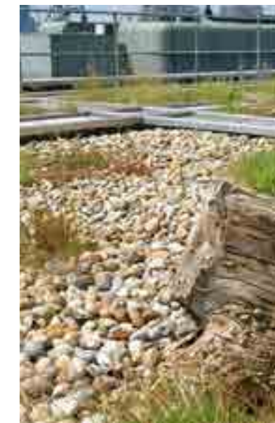
Varied surface and log piles on dry meadow roof
