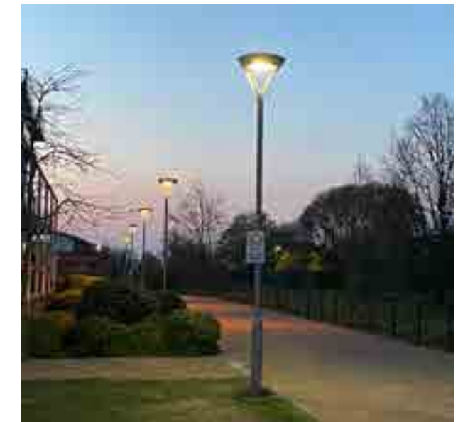
Pedestrian level lighting using low illuminance to minimise impact on adjacent wildlife corridor
