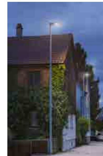
Lighting on a street with vehicular access. Credit: Igguzini
