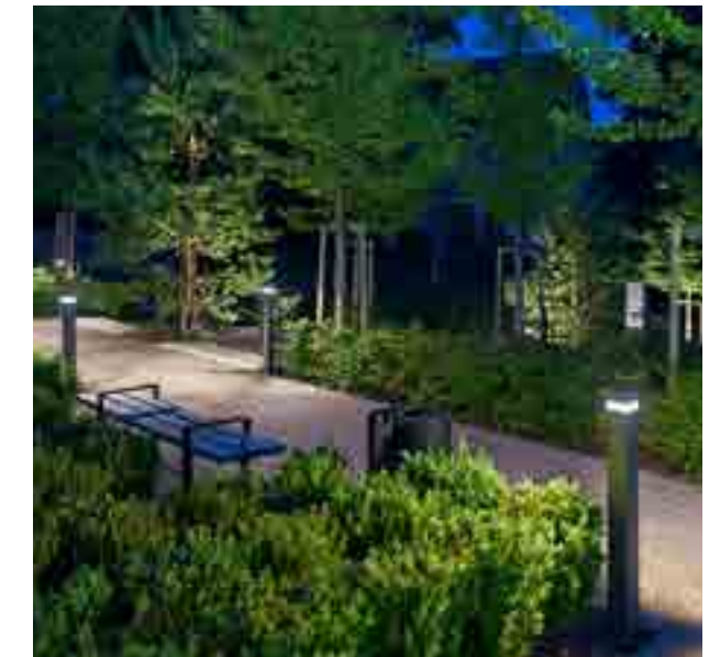
Low-level lighting should be used adjacent to wildlife habitats. Credit: Igguzini
