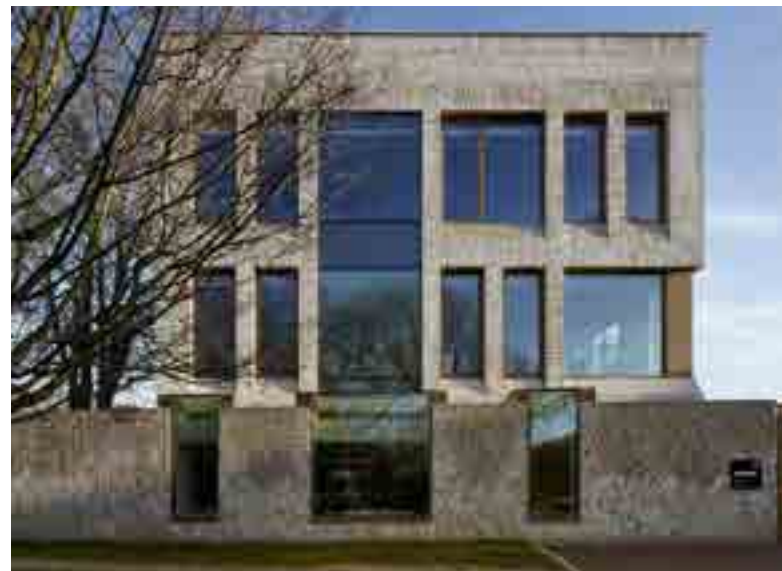
Imperial War Museum workspace (by Jestico + Whiles), constructed off-site using MMC. The building's triple-aspect workspace utilises natural ventilation and daylighting strategies, reducing energy demand on active systems. Photo credit: ©Matt Clayton
