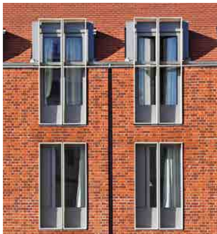
An uncluttered facade articulated through symmetry of elements including generously sized windows with deep reveals, recessed drain pipes and dormer windows. Brighton College Boarding House by Allies and Morrison. Photo credit: Fisher Hart.
