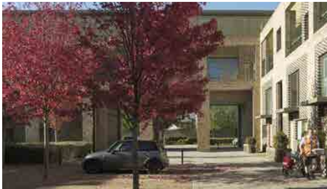
The impact of planting is mitigated by trees and planting. Credit: Proctor Matthews
