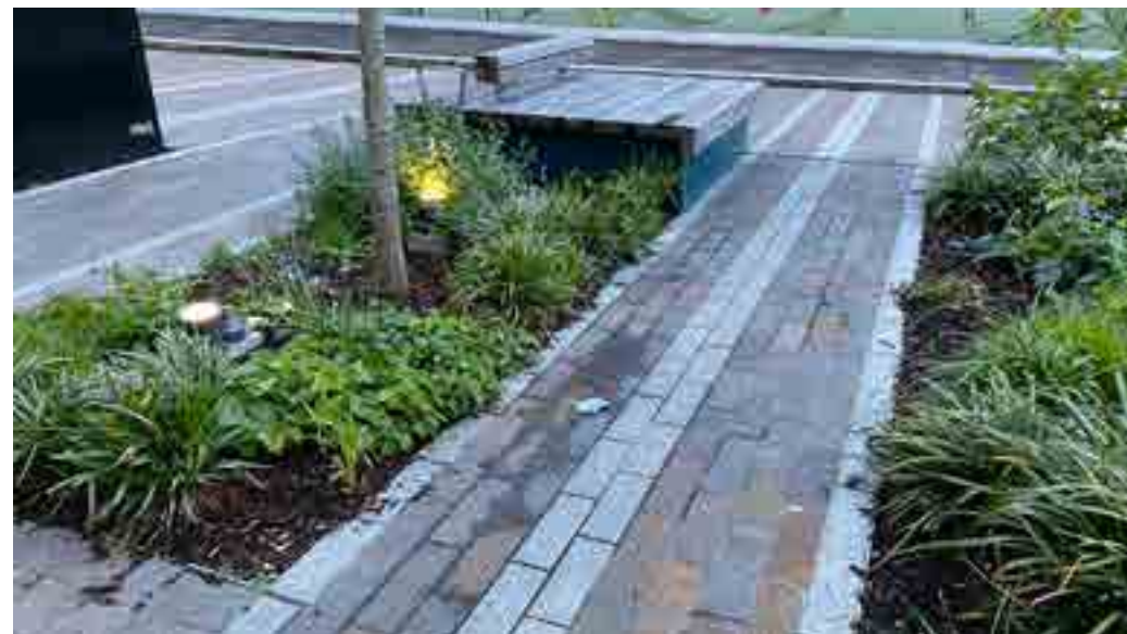
Example of high-quality and durable materials within a public square, integrated with planting and seating
