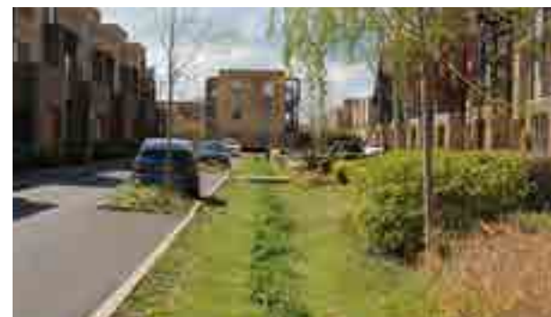
Street swale adjacent to car parking
